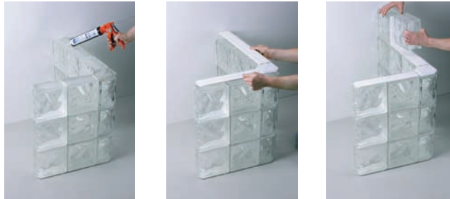
ProVantage® Glass Block Installation System using HEDRON® Corner Block.
